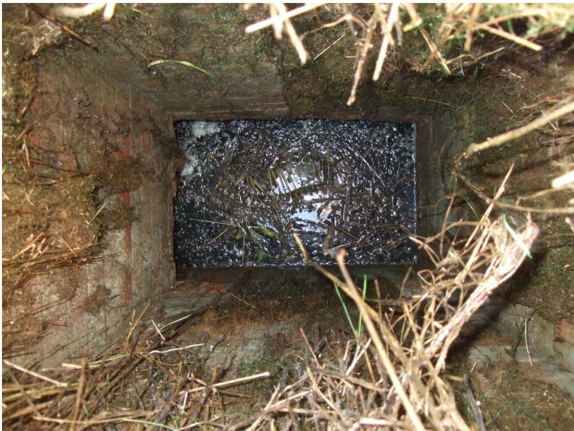
Photograph 14 Deep uncovered chamber in northern part of the site
