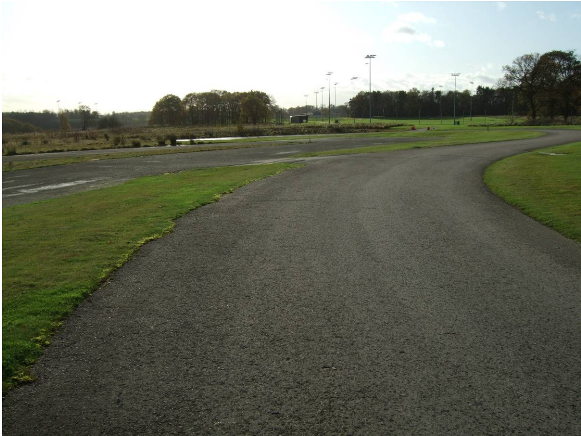
Photograph 3 Panorama from north west corner
