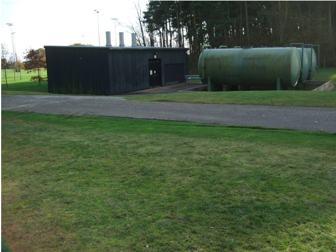
Photograph 15 Underpitch heating building and fuel tanks to west of site
